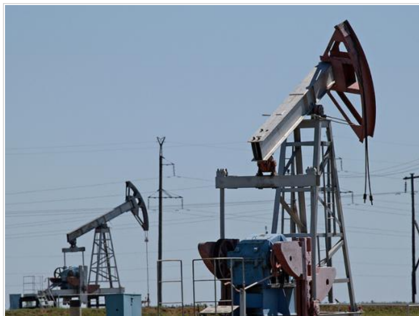
Oil pumps, in southern Russia. Photo: Gennadiy Kolodkin / World Bank
