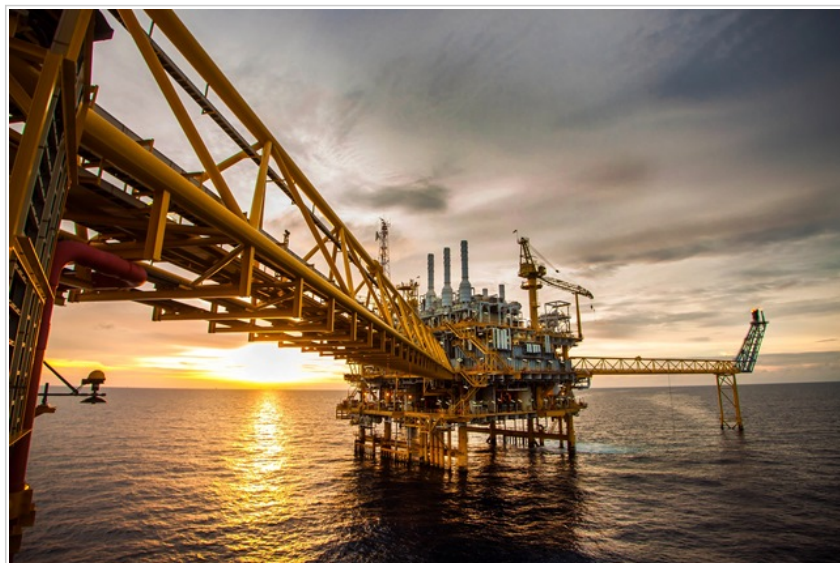
Offshore oil and rig platform. Photo: © curraheeshutter / Shutterstock.
